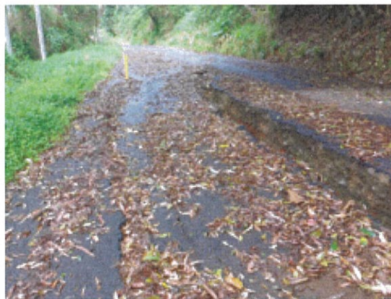
Figure 2 - Longitudinal settlement in road
